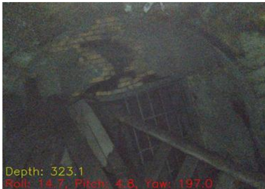
Figure 45 The entrance to the 306 m side passage is in shaft 10. The depth in the picture differs from the actual depth due to the difference in water density.
