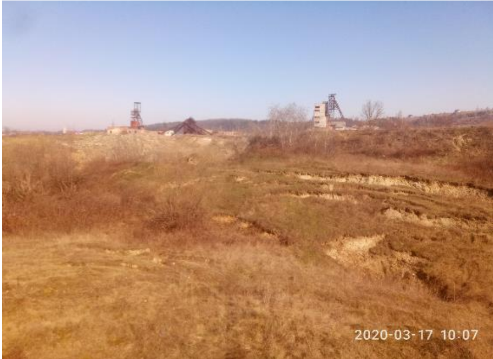
Figure 3 C. Trough-shaped subsidence zone complicated by karst sinkhole near the southern slope near the railway bank (Photo 2020-03-17)
